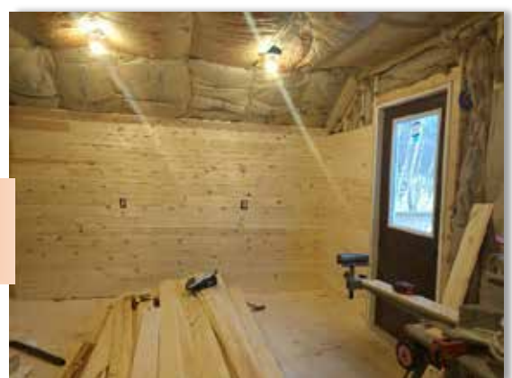
PANELING THE WALLS OF THE BUNKROOM
