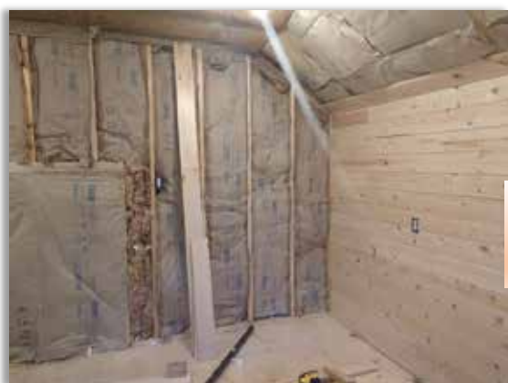
PANELING THE WALLS OF THE BUNKROOM
