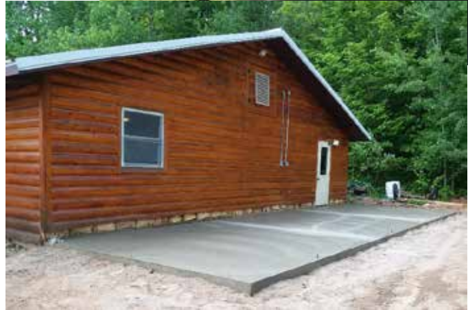
Pouring the slab for the cafeteria addition
